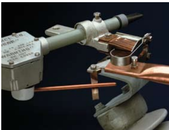
The arcing horn will pick up load current upon closing to prevent burning or arc pitting on the main contact surfaces.
