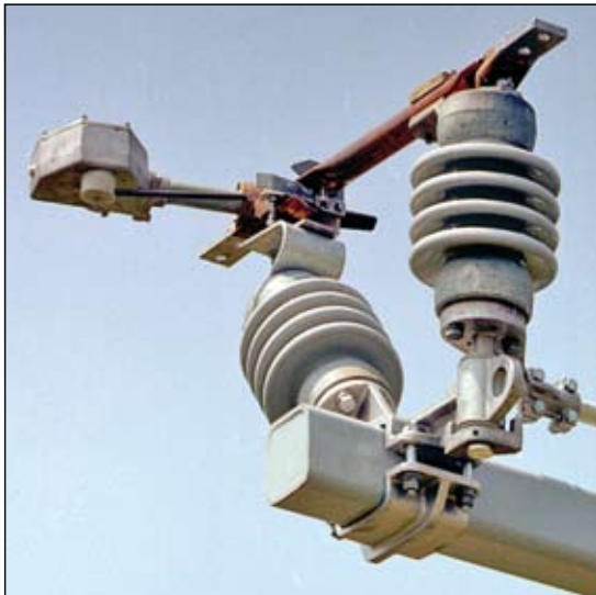
Chance 15.5, 27 and 38 kV Duogap expulsion interrupters .
